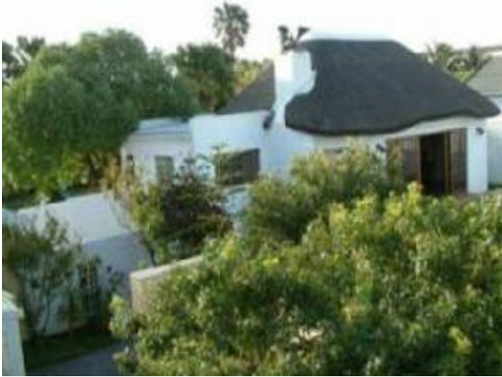
General house view
